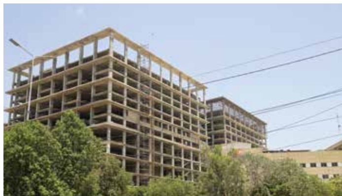
100% GREY STRUCTURE OF HB 1, HB 2 & IUHS COMPLETED
